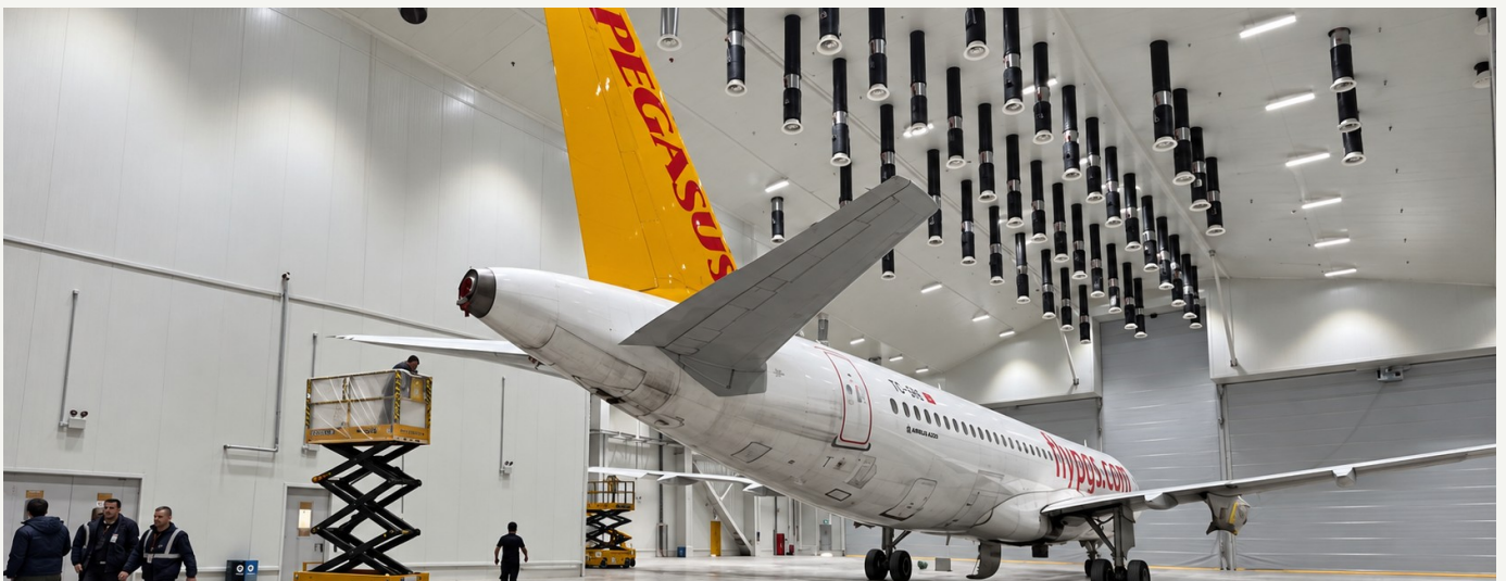
Pegasus Airlines aircraft paint hangar
