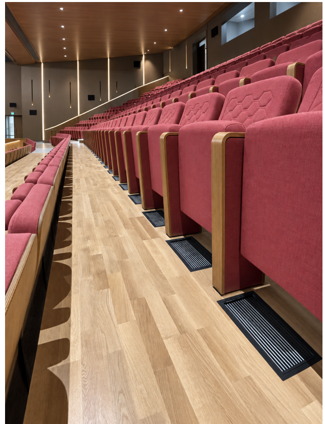
Figure 10. Under-seat displacement ventilation.
